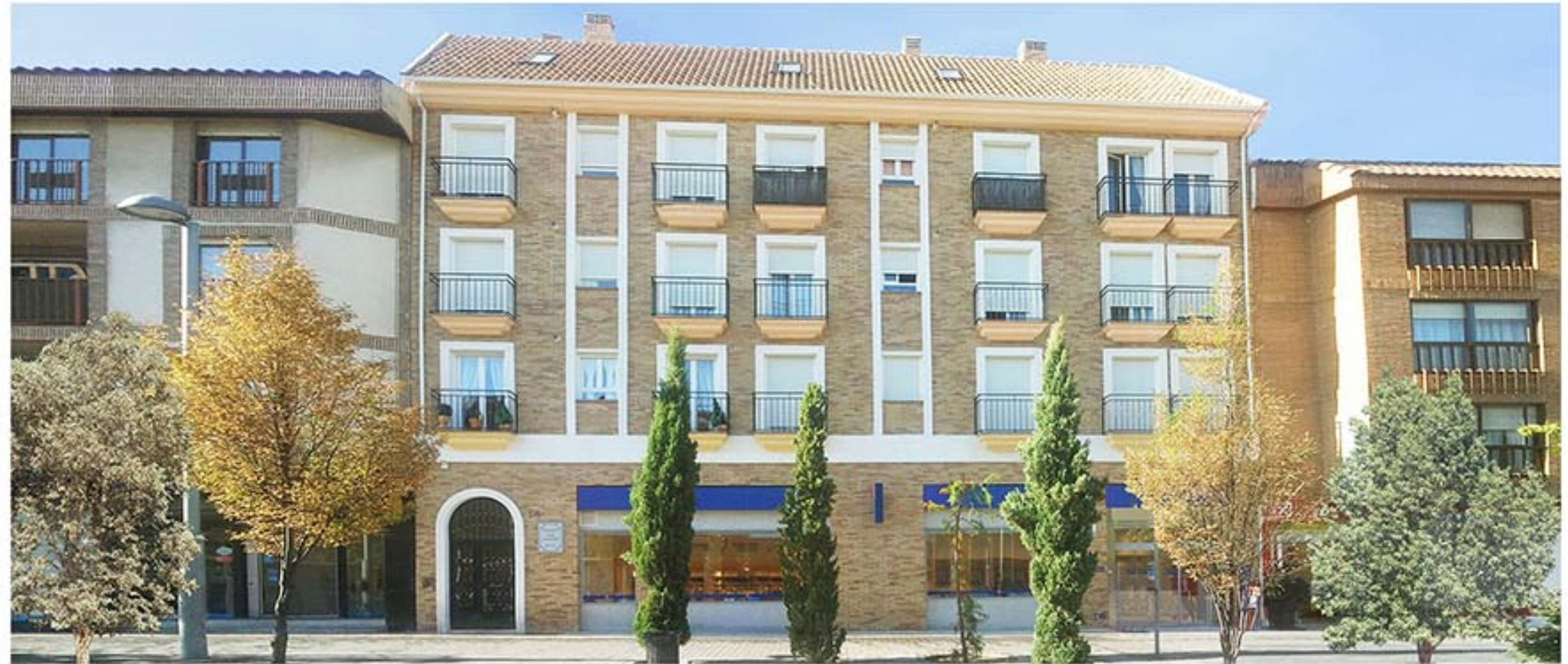
27-Unit Apartment Building in Las Rozas - Madrid
